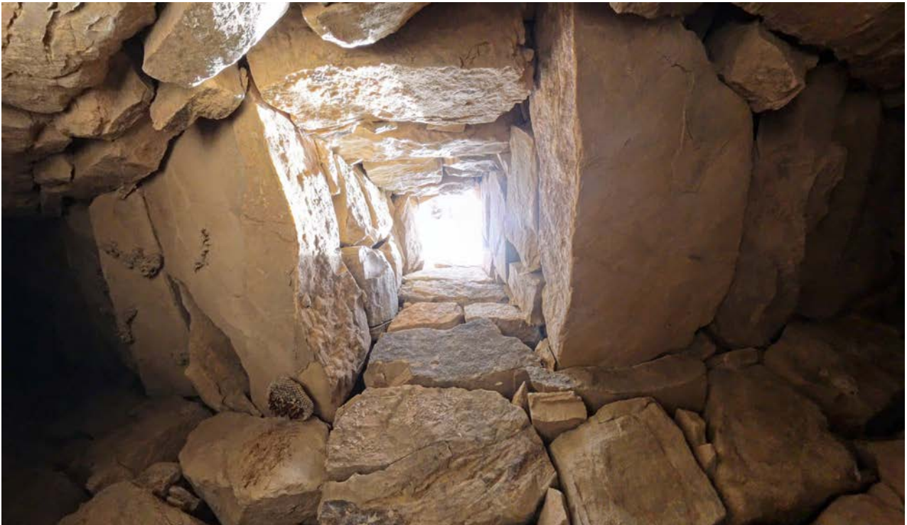
Figure 5. Internal view of a well preserved shaft made of stone stone bricks along the falaj of Figure 4.
